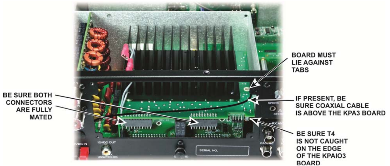
Figure 24. Reinstalling the KPA3 Module.
